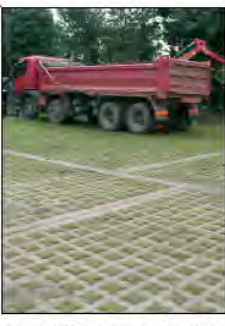
TYPICAL GRASSCRETE PAVING AFTER INSTALLATION
