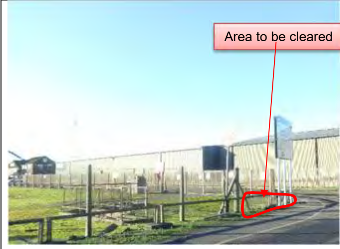
8.4.2.3. – View at crossing
